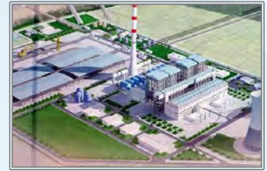
Hung Yen Thermal Power Plant
