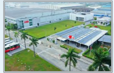
ABB Factory Bac Ninh, Vietnam
