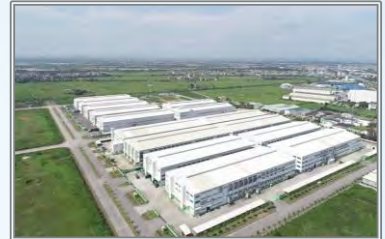
Centralized Wastewater Treatment Plant An Phat 1 Industrial Park
