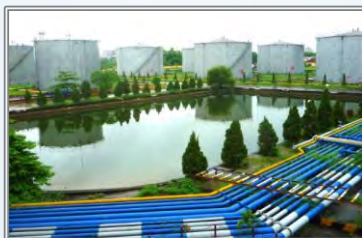
Southeast Duc Giang Oil Depot Hanoi
