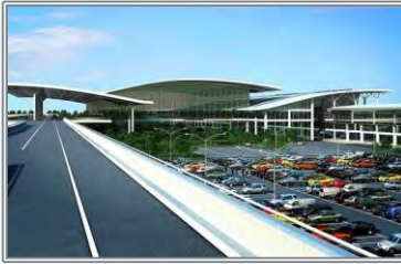
Noi Bai International Airport
