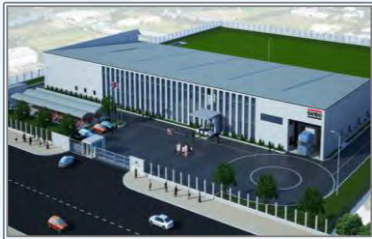
BANDO Vietnam Manufacturing Plant
