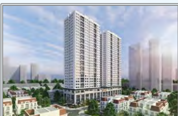
ICID Complex Building Ha Dong - Hanoi
