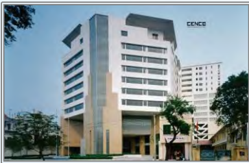
Renovation Sun Red River Building Hanoi
