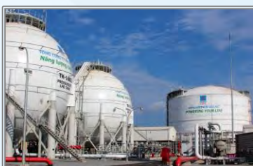
MMPA LNG Storage Warehouse 1 Thi Vai Port ,Vung Tau
