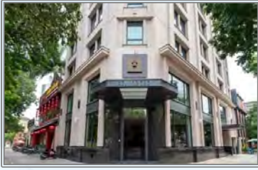
VIE building 28A Tran Hung Dao
