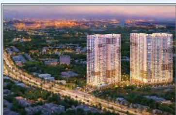
Opal Boulevard Building Binh Duong
