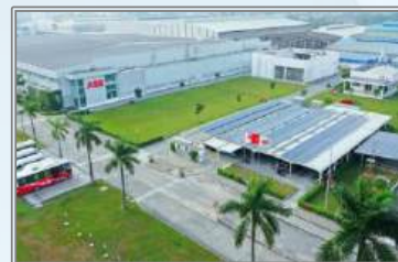
ABB Factory Bac Ninh, Vietnam
