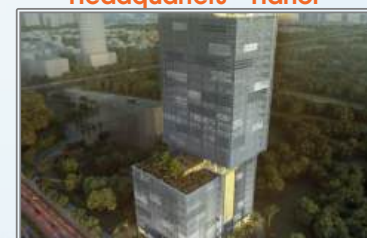
Headquarters Building of the Telecommunications Bureau - Hanoi
