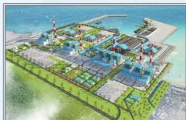
Vinh Tan 1 Thermal Power Plant Binh Thuan
