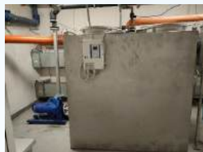
Automatic Grease Separators use an automatic controller, valve and pump
