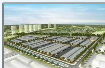
Mapletree Logistics Warehouse Bac Ninh
