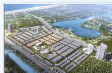
Bau Tram lakeside Danang
