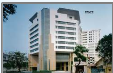
Renovation Sun Red River Building Hanoi
