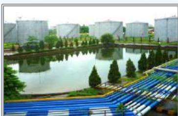
Southeast Duc Giang Oil Depot Hanoi
