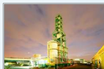
Tan Binh Chemical Factory 2 Dong Nai
