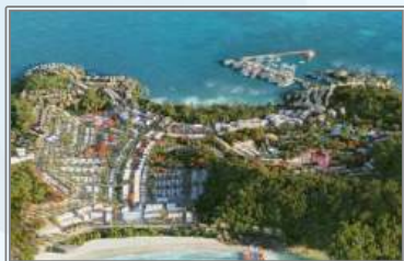
Shophouse Western Village Hon Thom, Phu Quoc
