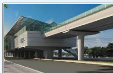
Metro Station Hanoi
