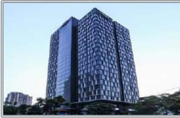
Vinaconex 34 Office Building - Hanoi
