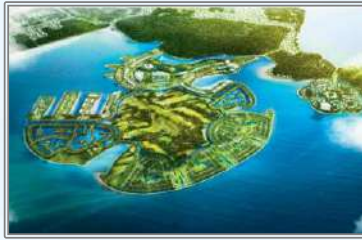
Dragon Hill Project – Hai Phong
