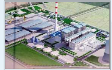
Hung Yen Thermal Power Plant
