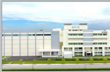
Rorze Robotech factory Hai Phong
