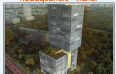
Headquarters Building of the Telecommunications Bureau - Hanoi
