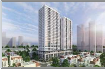
ICID Complex Building Ha Dong - Hanoi
