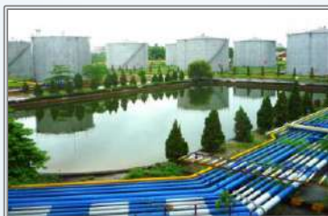
Southeast Duc Giang Oil Depot Hanoi
