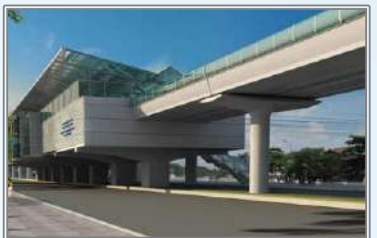
Metro Station Hanoi
