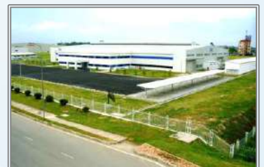
Vietnam FCC Factory Thang Long Industrial Zone, Hanoi
