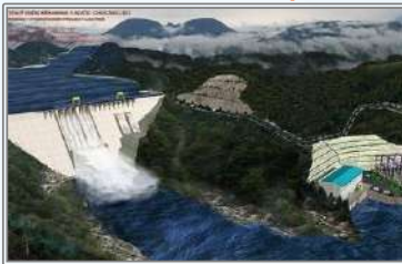
Hydropower Plant Xekaman 1 - Lao
