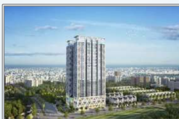
The Zei Building Le Duc Tho - Hanoi
