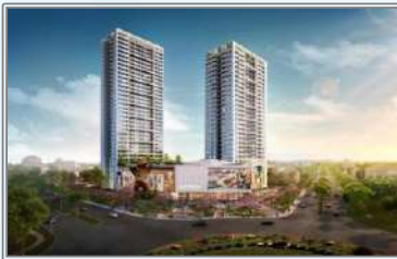
Vinhomes Bac Ninh
