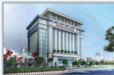
State Bank of Vietnam Headquarters - Hanoi
