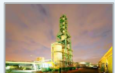
Tan Binh Chemical Factory 2 Dong Nai
