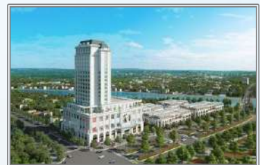
Renovation of the Ministry of Public Security Headquarters - Hanoi
